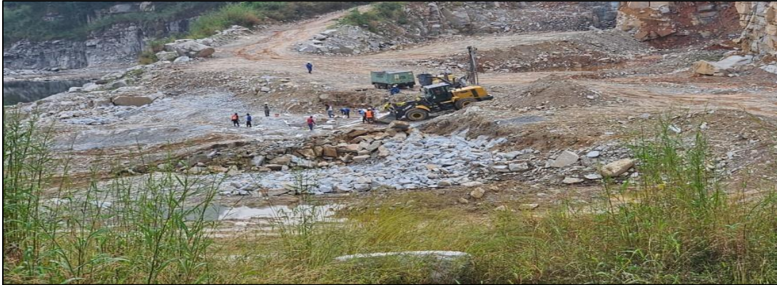
Figure 2 Drilling machine on site
